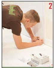
Mark the holes with a pencil while holding the StepNpull® against the door in the appropriate level mounting position. If a metal kick plate is on the door, drill 6mm holes, where marked for the bracket, through the metal plate before going to the next step (only go through the metal and be careful not to drill into the door).
