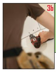
Metal doors: Drill a pilot hole for each of the three holes using a 5mm bit. A sexed bolt should be used in the middle hole and 30mm long screws in the outer two holes. To prepare the centre hole for the sexed bolt, use a 8mm bit to enlarge the centre hole and then continue drilling through the outer metal skin (be sure to keep the drill bit perpendicular to the door while drilling the outer hole). Remove any burrs. Loctite thread locker should be used on the bolt threads.
