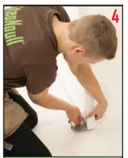
Hold the StepNpull® against the door and install the centre screw/bolt but don't tighten it completely. Install the two outer screws. Tighten the centre screw and then double check the outer screws. To avoid stripping the screw head, use a large #2 or #3 Phillip's screwdriver or bit.
